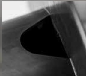
7. This cut-out allows the cable to be close to the flange.
